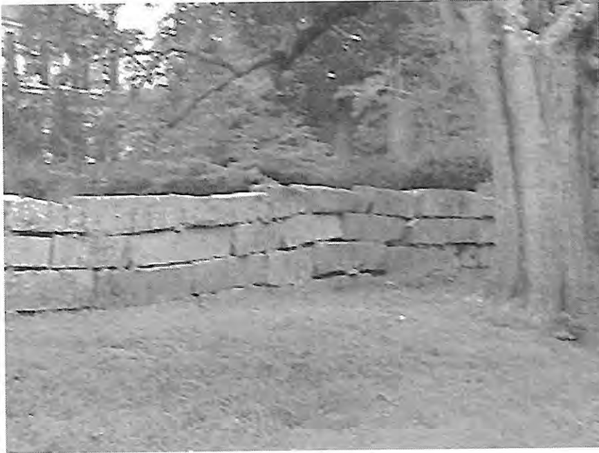
Stacked, semi-dressed granite wall
