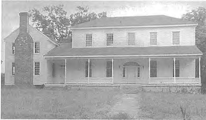
Left: The Lumpkin-Maxwell-Montgomery House, ca. 1790's, is an early vernacular I-House (seen on the left) with a Federal Style wing added around 1827. The porch is a later Victorian addition.
