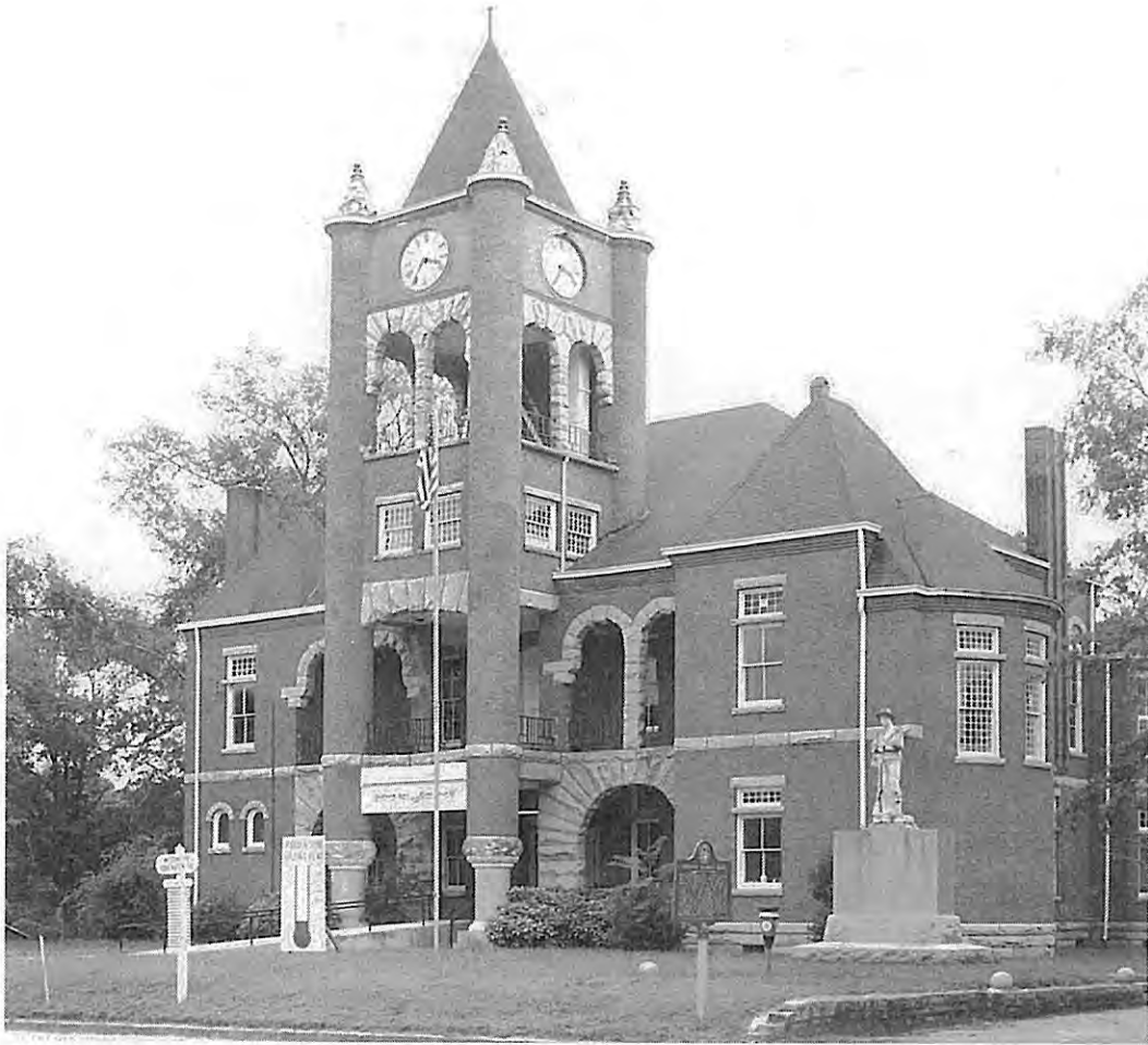
The Oglethorpe County Courthouse, ca. 1886, an imposing brick and granite building with an elaborate central clock tower, granite framed arches, and ornamental limestone and terra cotta, is a fine example of the imposing Richardsonian-Romanesque style, favored for important government buildings in the 1880s-90s.
